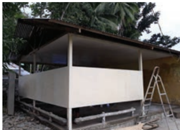
Temporary Learning Spaces in construction, facilitated by DepEd
