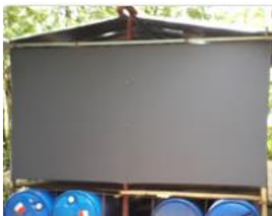
Figure 19: Floating Store room under construction
