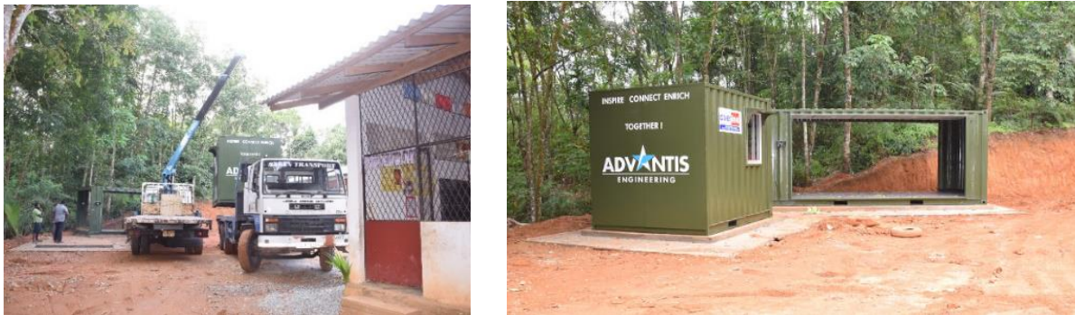
Figure 20: Positioning converted containers for store and kitchen
