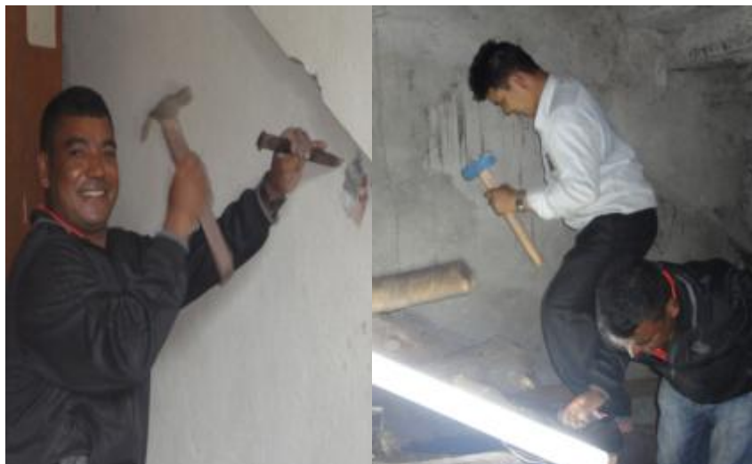
Figure 5-1 Surface preparation works
