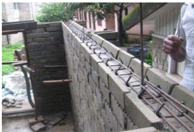
13. Reinforcement for Lintel
