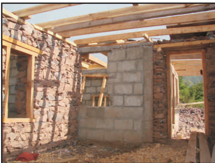
Never mix different masonry materials at the same level in a building.
