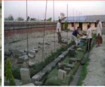
6. Laying of blocks
