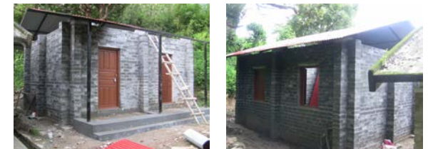
Figure: Completed Structure of CSEB
