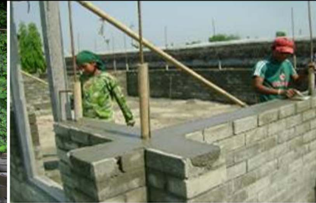
11. Concreting of Sill Band
