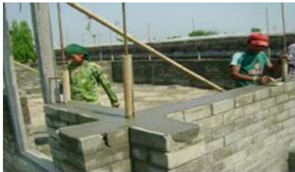
11. Concreting of Sill Band
