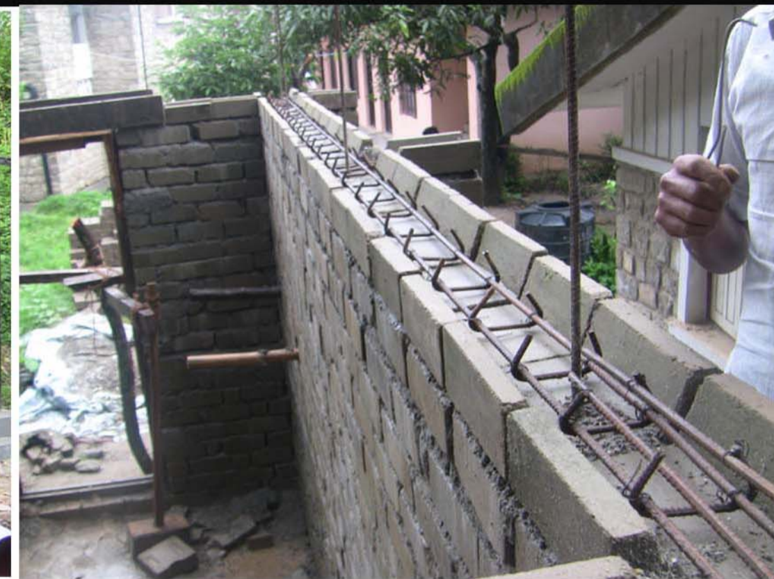
13. Reinforcement for Lintel
