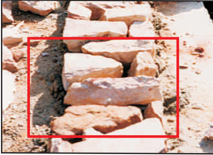
Break all vertical and horizontal joints in masonry
