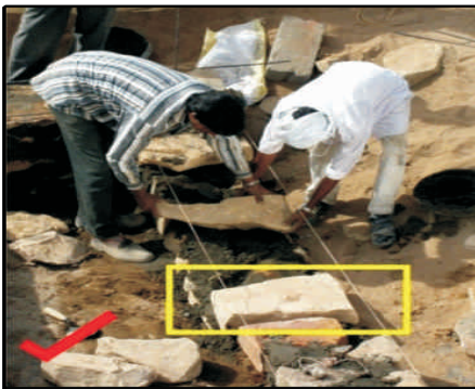
Provide "through-stone" one in every 0.7 sq.m. and arrange in zig-zag pattern.
