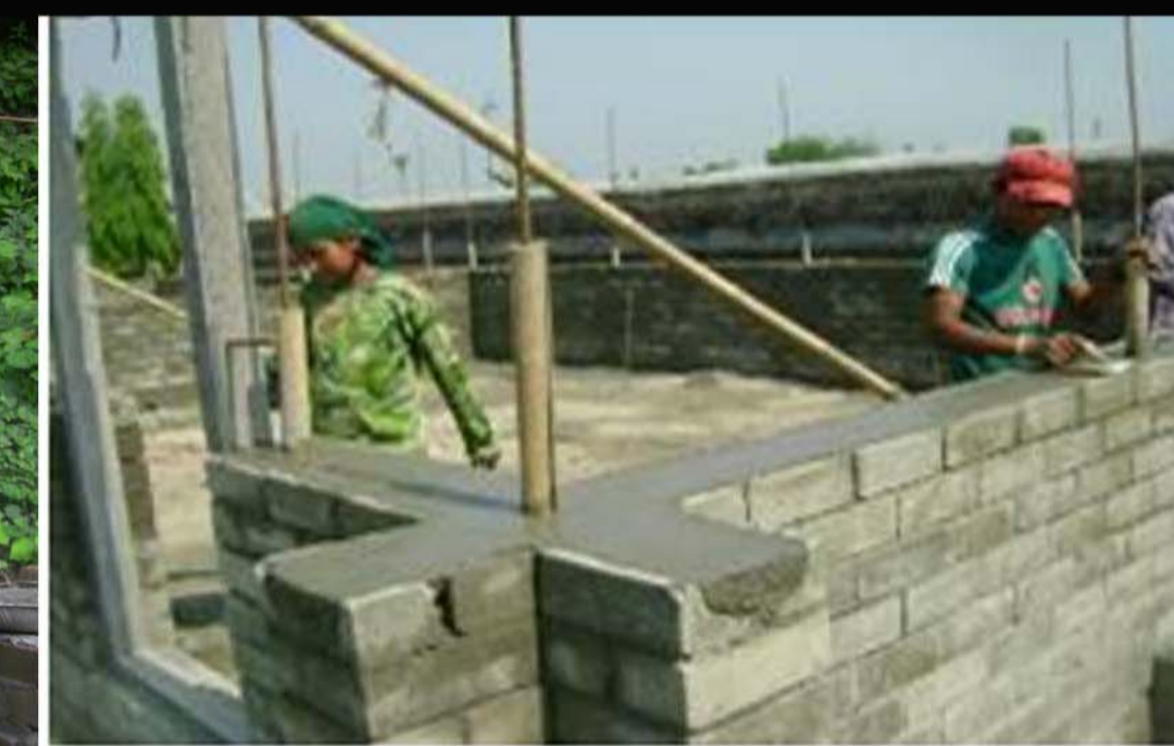
11. Concreting of Sill Band
