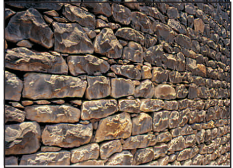
Break all vertical and horizontal joints in masonry
