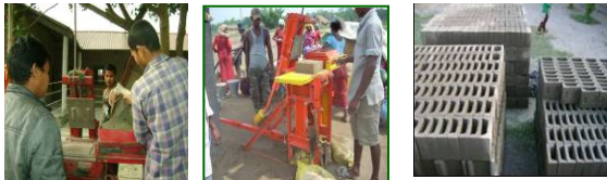
Figure: Moulding, storing of CSEB
