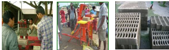
Figure: Moulding, storing of CSEB
