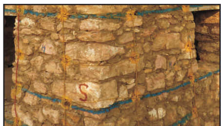
Earthquake Resistant House with GI wire Containment Reinforcement
