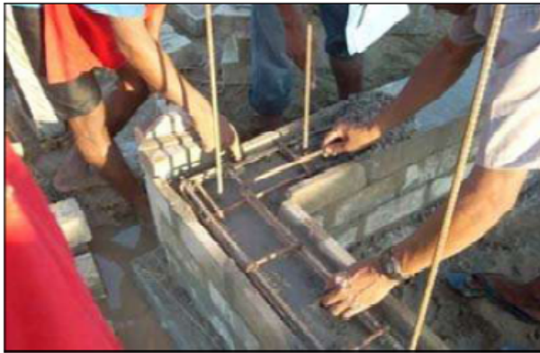
Connection between enn walls
