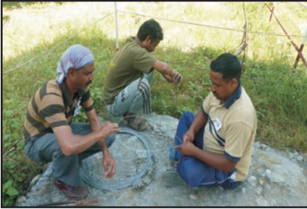
Making GI wire cross links.
