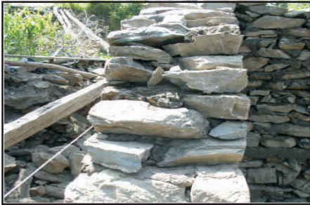
Place each stone flat on its broad face.
