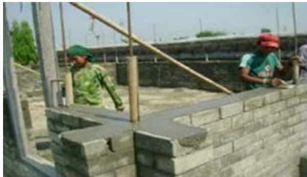
11. Concreting of Sill Band
