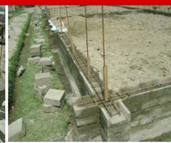
7. Reinforcement in plinth beam
