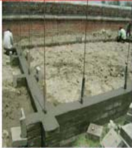
8. Completed Plinth Beam
