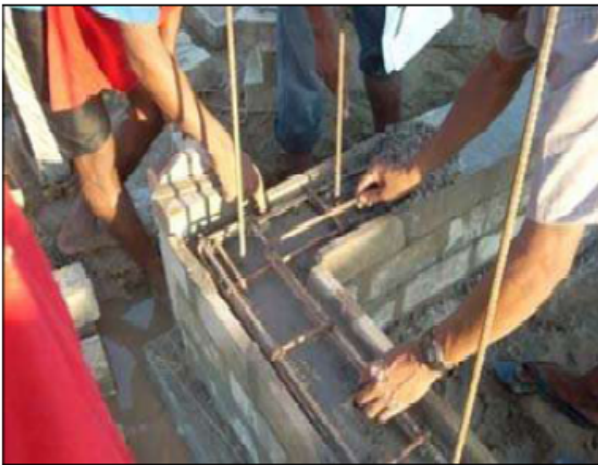
Connection between enn walls
