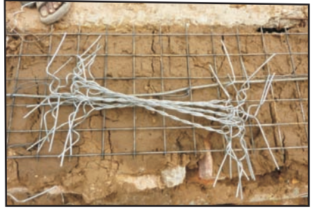
GI wire cross links with open ends .
