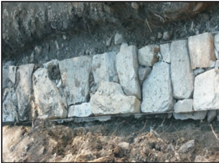
Orient length of each stone in to the thickness of wall to ensure interlocking of inside and outside faces of wall.
