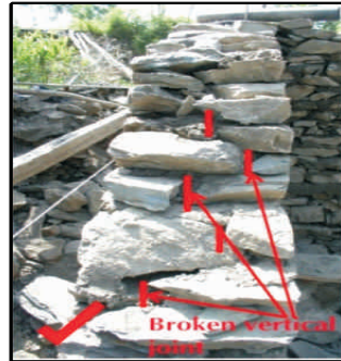
Both faces must lock with each other to form one wall. Vertical joints must break.
