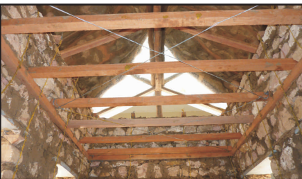
Earthquake Resistant House with GI wire Containment Reinforcement
