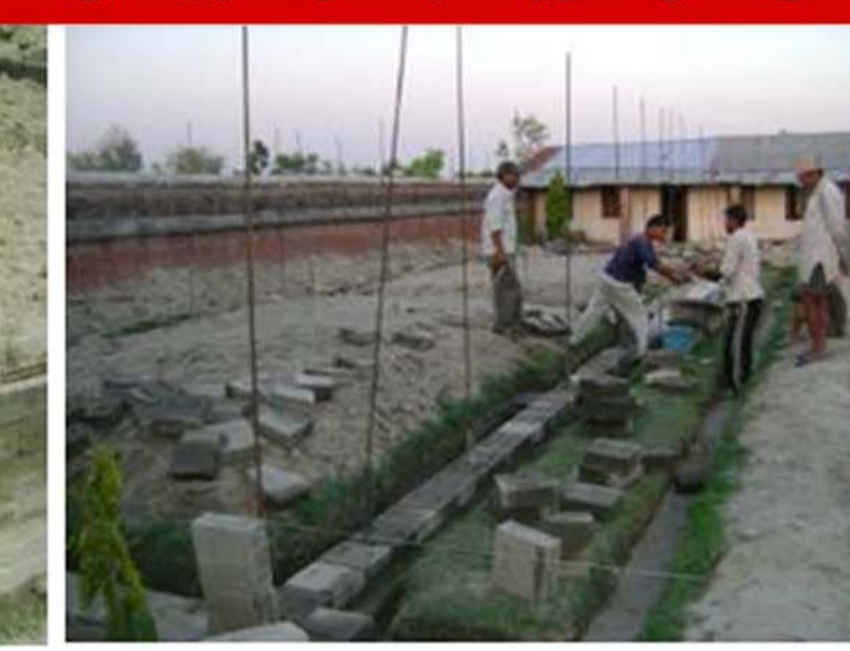
6. Laying of blocks
