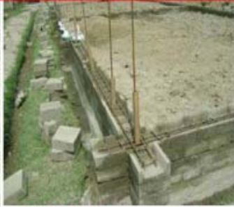
7. Reinforcement in plinth beam
