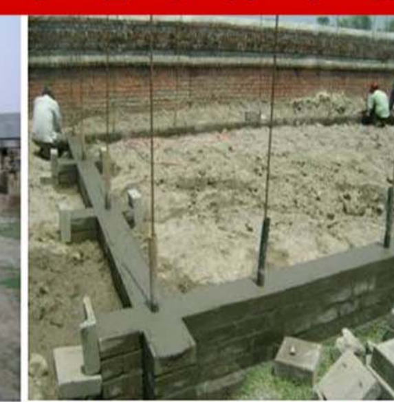
8. Completed Plinth Beam
