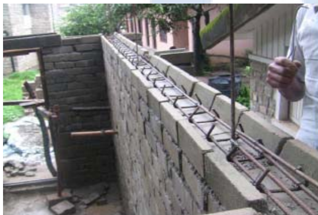
13. Reinforcement for Lintel
