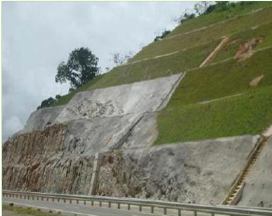
Figure 2-2 Slope protected with berm drains, cascade drains and surface protecting measure
