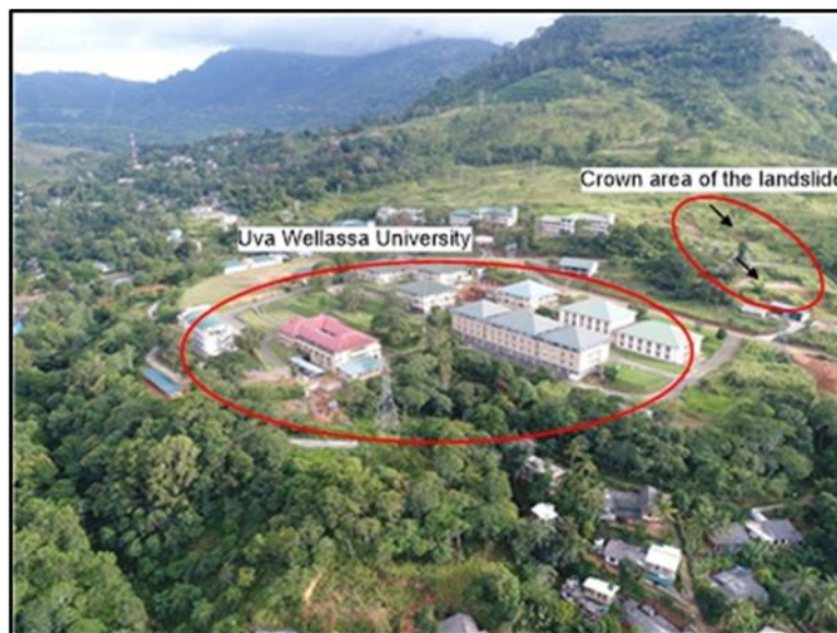
Figure 4-2 Aerial view of upslope of the landslide and Uva Wellassa University Premises
