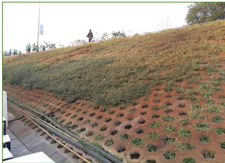
Figure 11-9 An example of Hollow Block vegetated cover in a slope in Vientiane, Lao
