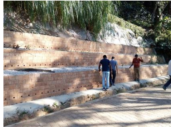
Figure 11-5 Appearance of a TOR Block Wall system with space for bench planting. Chiang Rai, Province, Thailand
