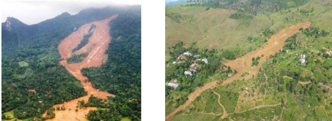
Figure 1-1 Debris Flow - Landslide at Aranayake (a) and landslide at Meeriyabadda (b) (Dulanjalee, 2018)
