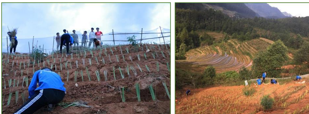
Figure 11-1 Vetiver grass planting in North- South expressway – Vietnam
